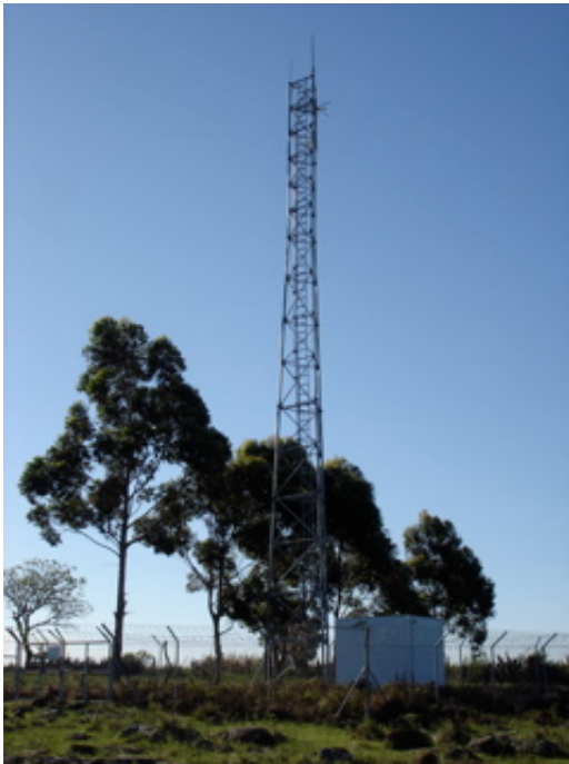
Figure D-4 Eskom tower relay station
