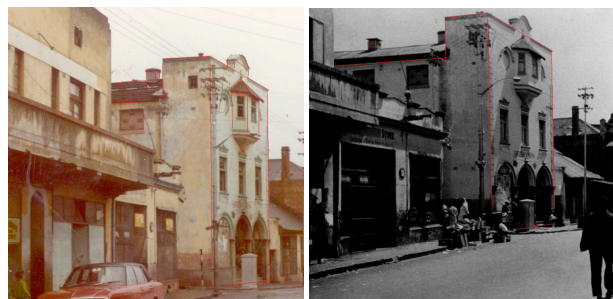
Figure 7: Photo input for the British Bioscope. Note the poor viewing angle with respect to the front wall, and the obstructions present in both photographs.
