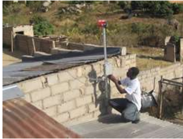
Figure 3 Community members are used to install the Cantennas. The Cantennas will connect rural areas like these to the world.
