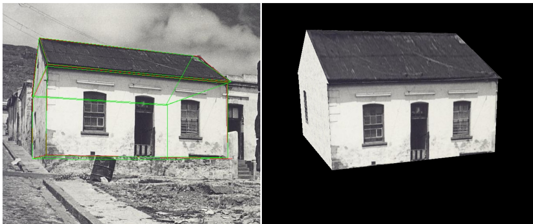
Figure 1: The original photograph is annotated to create a three dimensional virtual building
