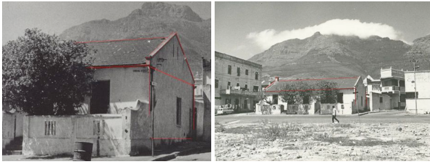
Figure 5: Photo input for a Large District Six residence. The relevant edges of these photographs have been marked out in red by the user.
