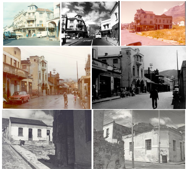
Figure 2: Some examples of the District Six photographic material. [Top] three photographs of the Hanover Building, a local landmark. One of the photographs is in greyscale, while another was taken during the demolition of District Six. [Middle] two photographs of the British Bioscope — a building we go on to reconstruct in Section 5. Again, one image is in greyscale, while the second is in colour. [Bottom] two images of different District Six buildings, for which we were unable to find additional, matching photographs
